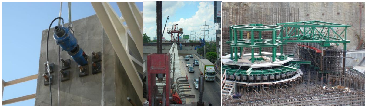
PT - Saadiyat Bridge, Abu Dhabi Beams lifting, Thailand Nuclear reactor, China
