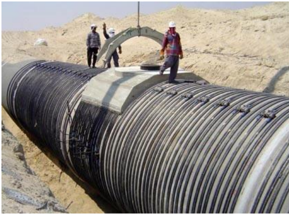
500km Pipe Repairs - Libya
